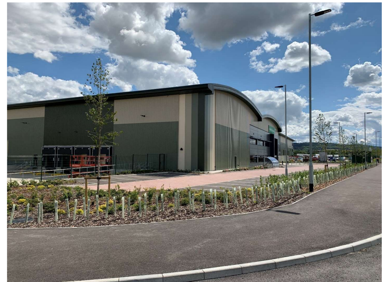
Fig 306. Column mounted and building mounted, light fittings for the development plots and highways.
